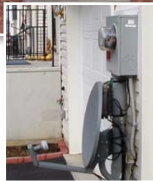
The satellite dishes shown do not allow proper clearance from the meter and transformer box above.
